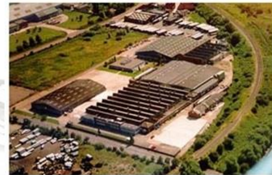
EnerSys Newport Facility Newport, Wales, United Kingdom
